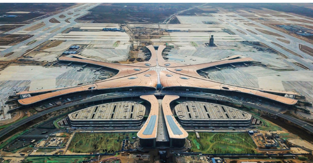
Beijing Daxing International Airport, China
