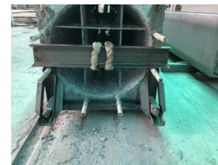
柱顶、柱底工装
